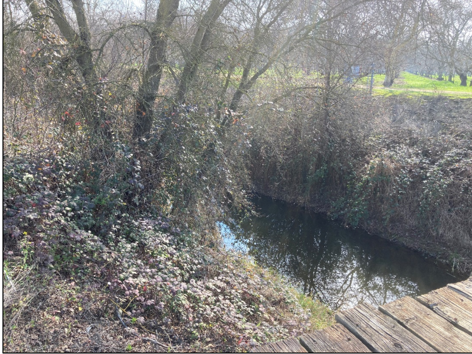
Photo 3. Representative of the disturbed riparian corridor and Calaveras River stream channel. Note the pattern of vegetation destruction which indicates the ordinary high-water mark of the stream channel (January 2021).
