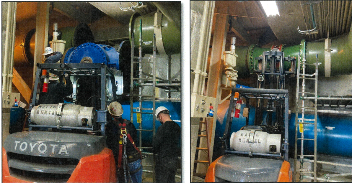
Figure 4. Master Backwash Valve Replacement
