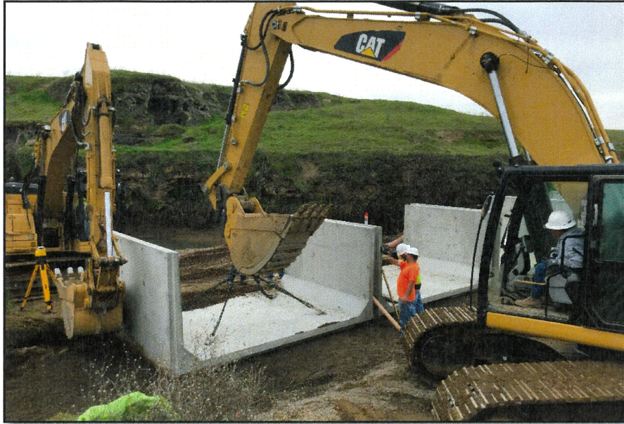
Figure 2. Whittle Ranch Main Crossing Construction
