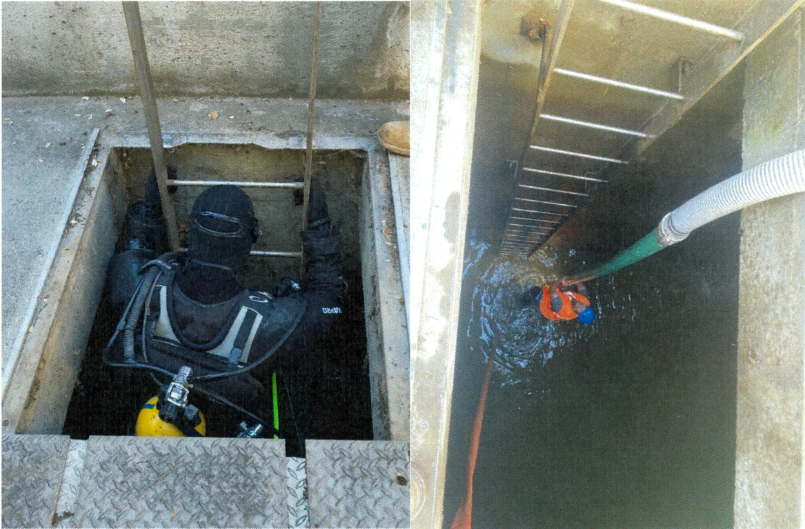
Figure 5. LLPS Sump Inspection and Cleaning
